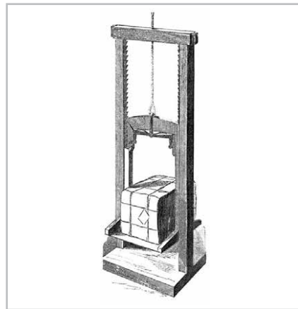
Figure 3 Elisha Graves Otis safety exhibited at the New York Crystal Palace (1854)
