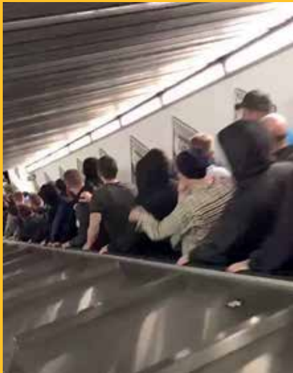
Photograph 2: Passengers during the initial phase of a runaway starting to hold the passenger in front.
