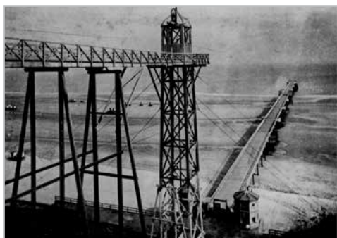
The original vertical lift
