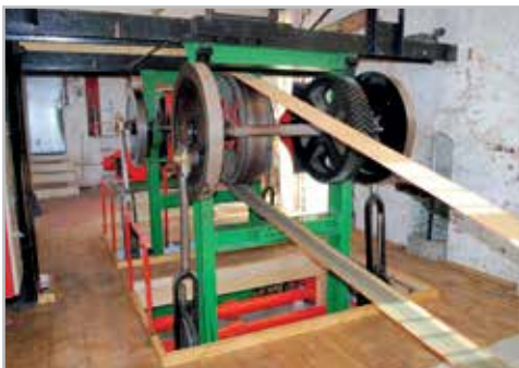
The pump room
