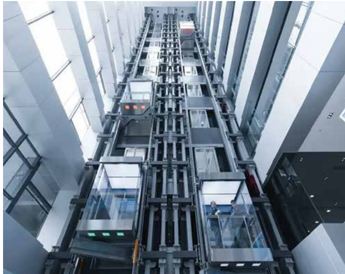
Figure 5. TWIN Elevator system shaft layout. © TK Elevator
